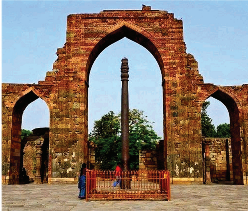
Figure 4. The stainless iron pillar of New Delhi, a UNESCO World Heritage Site. It is 7.2 meters high, 40 centimeters in diameter, weighs about 6 tons and is 1,600 years old.
